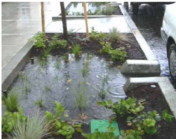
Stormwater planters along Hastings
