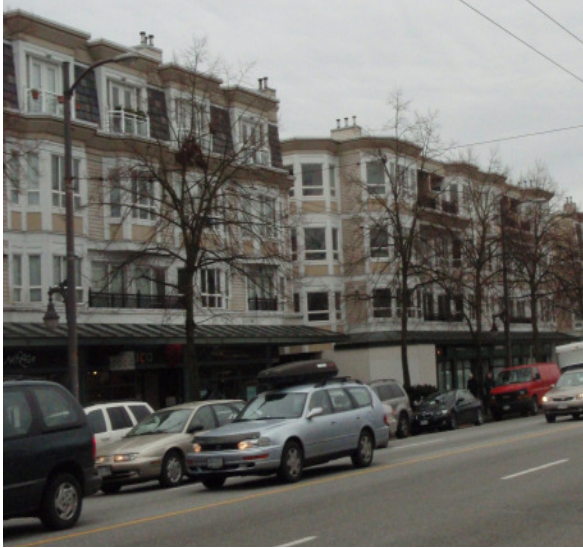
Four story building with commercial on the first floor
